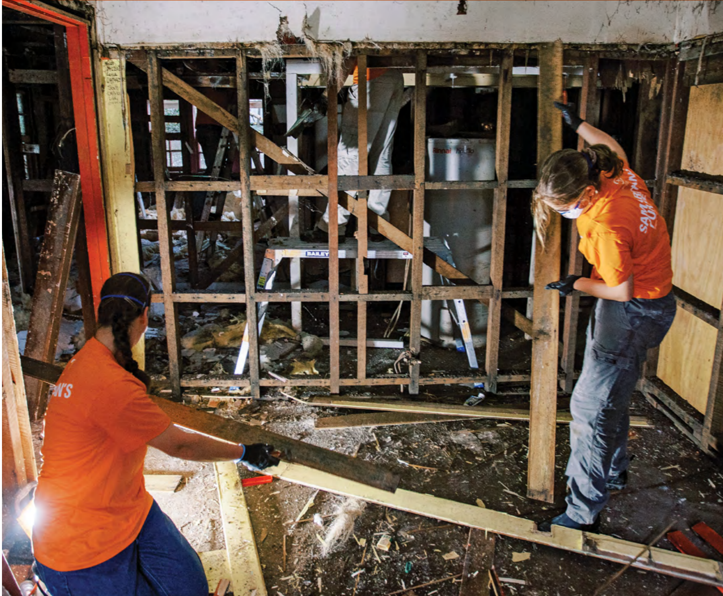
Stripping out flood damaged wall linings at Mirella's "Camp Davey", Lismore.
